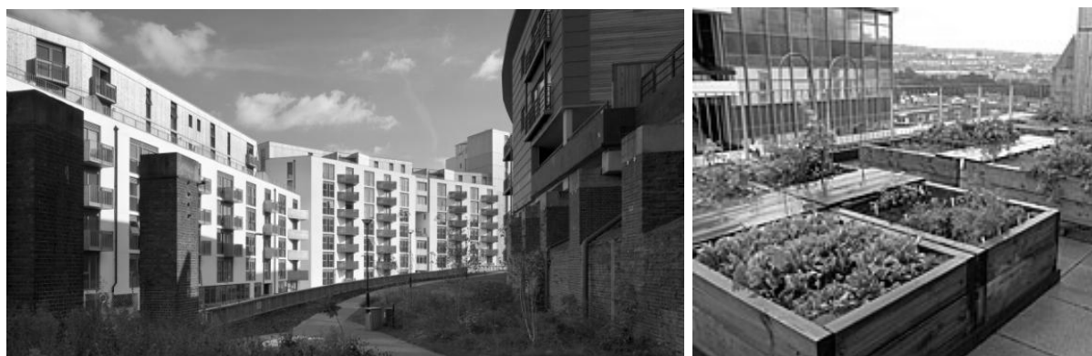
Figures 4 and 5. One Brighton rear elevation and roof top allotments.
