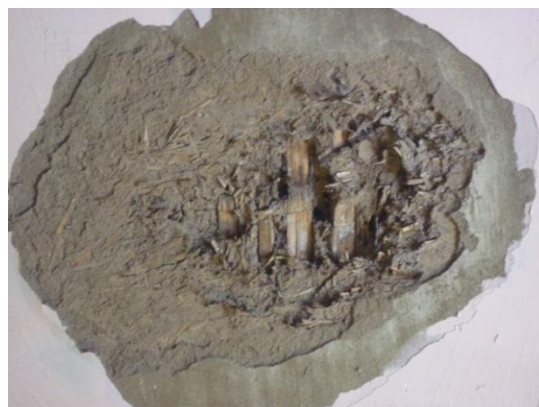
Figure 4:Detail of quincha wall build-up.
