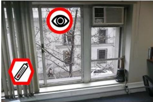
Figure 3: Example of recording visual and cold problems.
